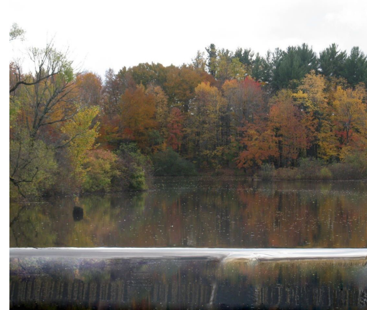
Fernwood Dam, Autumn 2015
