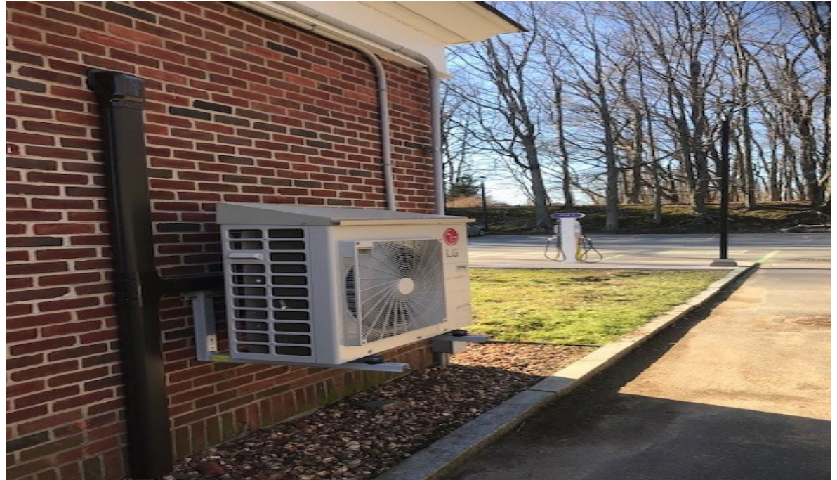
(Bottom) Heat pumps located in the library
