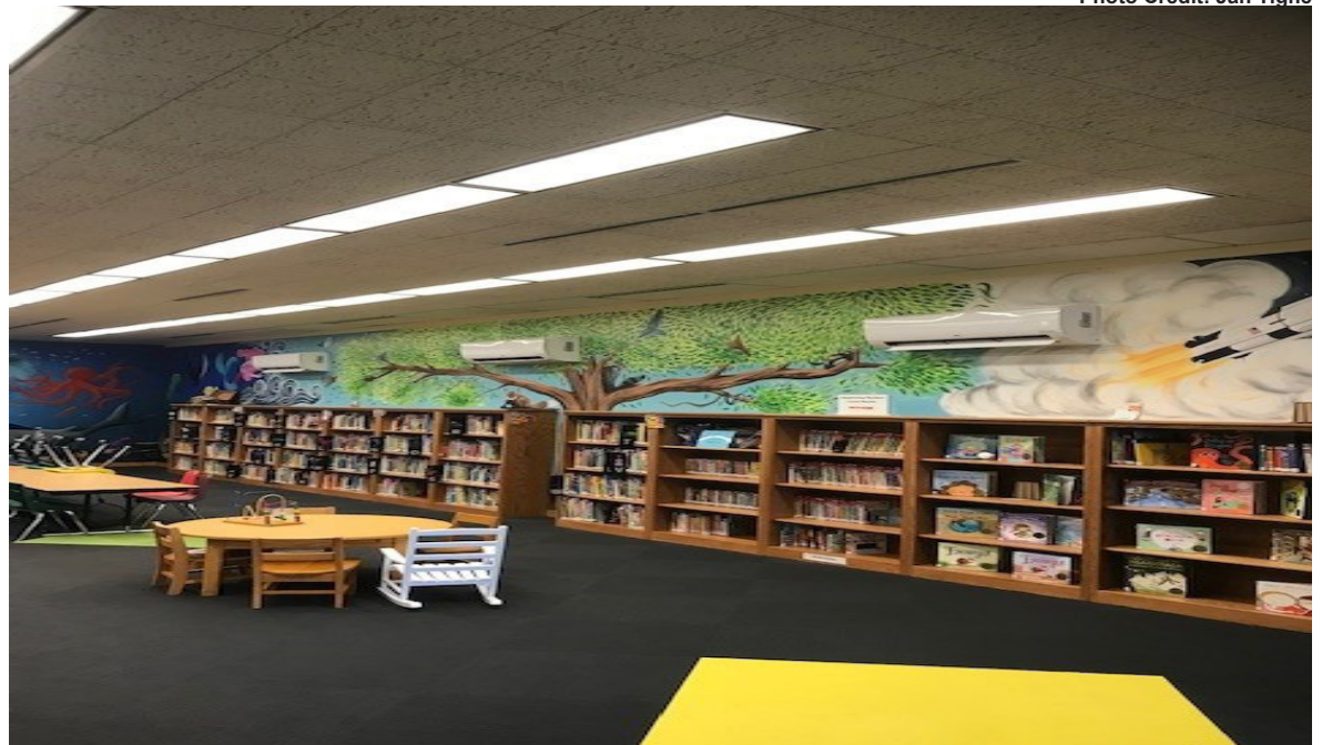
(Top) Air source heat pump installed at the Snow Memorial Building
